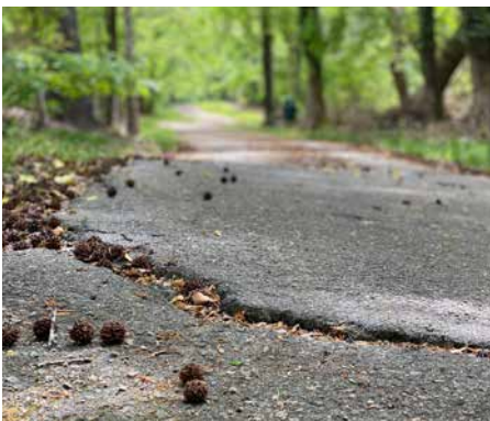
Image 35: Pavement Cracking
