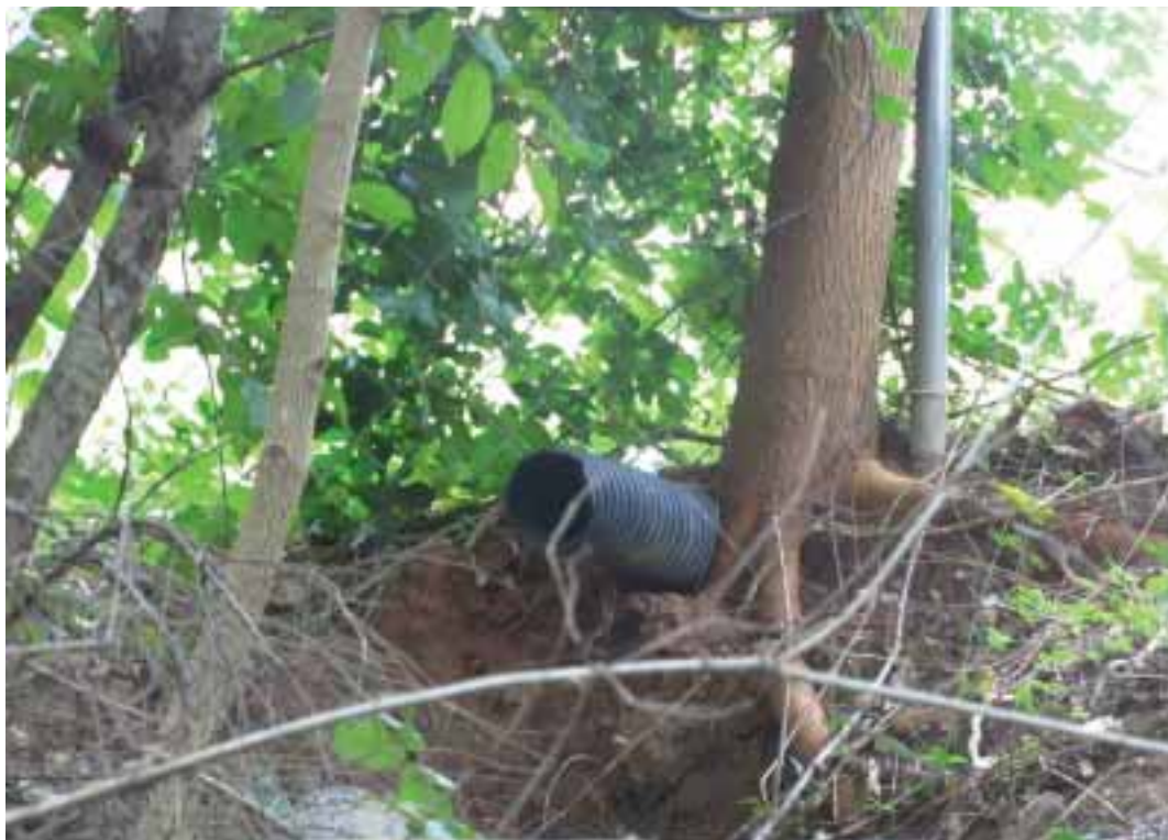
PVC pipe from multi-family housing unit, routing water to wooded stormwater draw. A section of chain link fence is located between the housing unit and woods.
