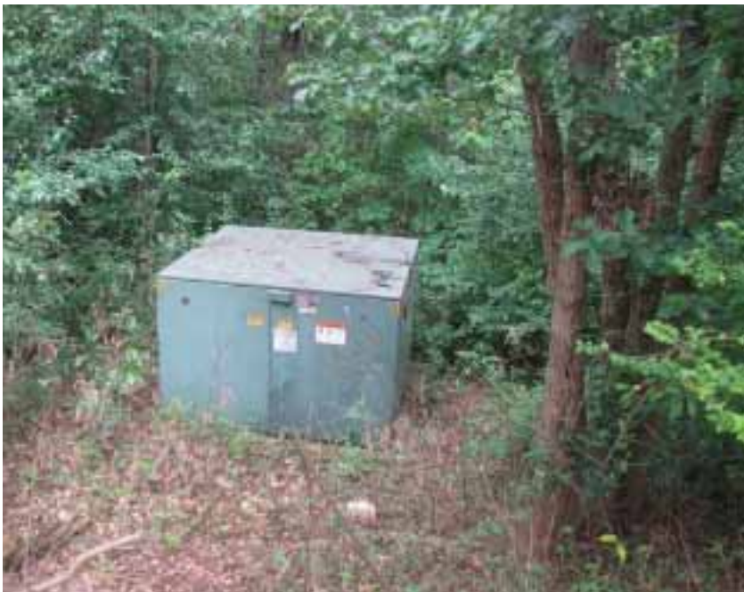
Large electrical transformer box in woods at southern corner of park property. This transformer box DIS No. 13086 is described in the Phase 1 ESA Report as unlabeled for PCB content.
