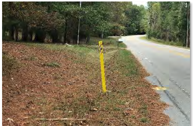
PSNC Gas Marker – Gas Line Location Is Evident Throughout Most Of The Project Area
