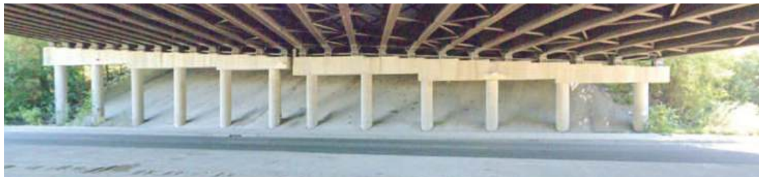
I-40 Underpass Along 401 (Top to Bottom)
