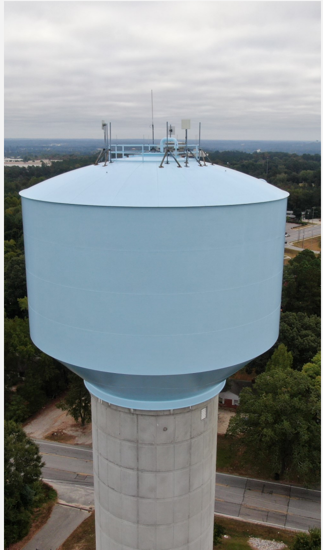
Reuse Water Tank on Sunnybrook Road
