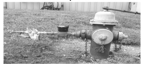
5/8" hydrant meter rental units are attached directly to the fire hydrant
