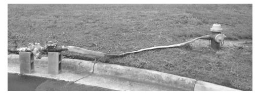
10' section of fire hose is provided by Raleigh Water for all 3" hydrant meter rental units. All customers that return 3" rental units with a bent hydrant connection port, due to a direct connection to a hydrant, will be charged for the replacement according to scheduled fees.
