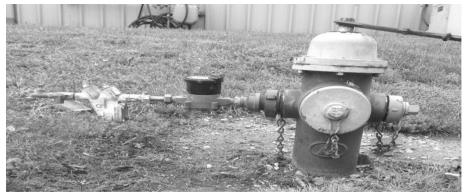
5/8" hydrant meter rental units are attached directly to the fire hydrant
