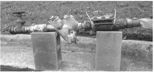
All 3" hydrant meter rental units must be stabilized a minimum of 12" above the ground to prevent debris entering the backflow assembly and to allow proper drainage
