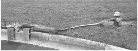
10' section of fire hose is provided by Raleigh Water for all 3" hydrant meter rental units.
