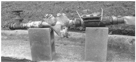
All 3" hydrant meter rental units must be stabilized a minimum of 12" above the ground to prevent debris entering the backflow assembly and to allow proper drainage
