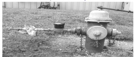
5/8" hydrant meter rental units are attached directly to the fire hydrant
