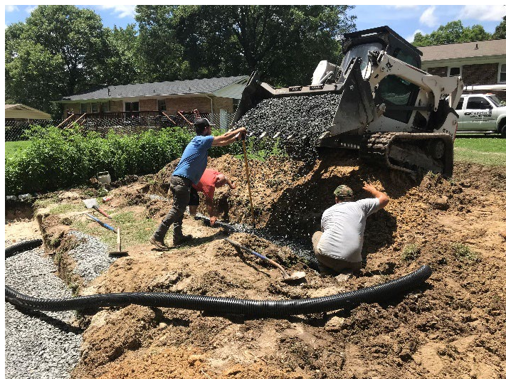
Figure 9: Installing new drainfield trenches at site with malfunctioning septic system (image courtesy of ECU EHSP)
