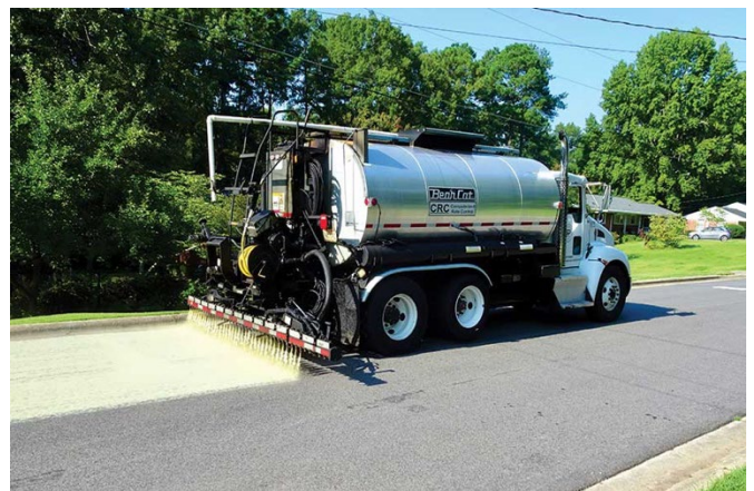
Image 16: City of Raleigh has been keeping cool! Cool roadways installation, like the one above, help the City of Raleigh reduce the impact caused by the Urban Heat Island Effect.
