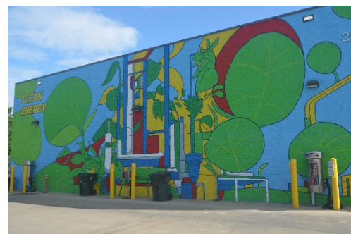
Image 26: Clean energy mural at the City’s Vehicle Fleet facility off Westinghouse Boulevard. This mural showcases the City’s continued priority of green energy.
