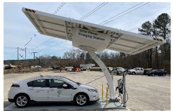
Image 12: Raleigh has rolled out its first set of Beam chargers! These chargers use energy from the sun to power the city's electric motor fleet.
