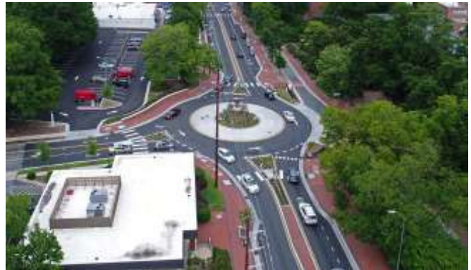
Image 6: Hillsborough Street roadway design to serve the needs of people walking safely and to calm vehicle traffic.
