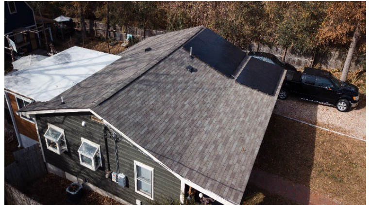
Image 4: Solar House installed through the Solar Pilot Program.
