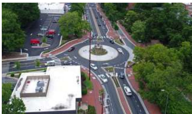
Image 6: Hillsborough Street roadway design to serve the needs of people walking safely and to calm vehicle traffic.
