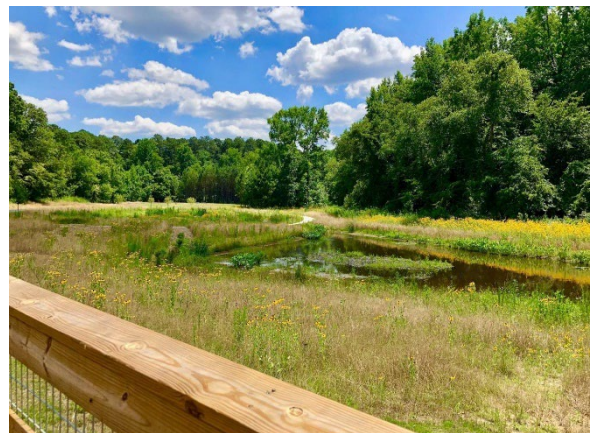
Figure 49. This constructed wetland is a type of green stormwater infrastructure. Raleigh Stormwater is committed to expanding green stormwater infrastructure (GSI) throughout Raleigh to reduce the community's exposure to flood hazards, lower energy consumption, create wildlife habitat, and reduce extreme heat in areas that most intensely experience these impacts.
