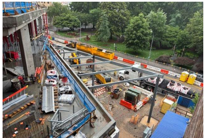
Figure 10. The construction contractor starts to install the Brise Soleil, a series of horizontal and/or vertical blades that help control the amount of sunlight and heat gain to a building. The Brise Soleil will shade the new City Hall terraces.
