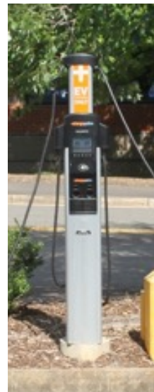
Figure 11. A Level 2 charging station on NCSU's Centennial Campus. Source: Advanced Energy
