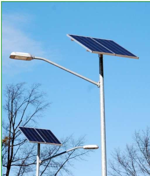
Solar LED Street Lights
