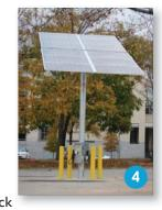
to Progress Energy. The two solar panels are a 2.88 kilowatt (KW) array combined, and are from different manufacturers to allow direct comparison of panel production. This is an example of a private/public partnership. (0.08 miles)
