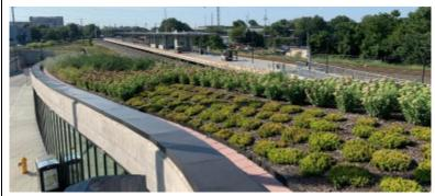
A green roof or living roof is a roof of a building that is partially or completely covered with vegetation and a growing medium. A green roof has many benefits: it provides a rainwater buffer, purifies the air, reduces the ambient temperature, regulates the indoor temperature, saves energy, and encourages biodiversity in the city.
