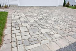
Permeable pavers allow water to soak into spaces in a hard surface. This reduces the amount of rainwater that runs off from hard surfaces into our streams and rivers, which can take with it harmful chemicals, trash and other pollutants. Water that soaks into the ground through the spaces between these pavers is filtered by soils, reducing the amount of pollutants in our rivers.
