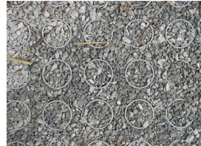
Photo 36. Close-up of vertical drainage pipes in crushed stone.
