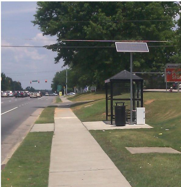
Photo 32. Well-equipped bus stop on Capital Boulevard include sidewalks, landing pads, shelter, light, trash can, and bench.
