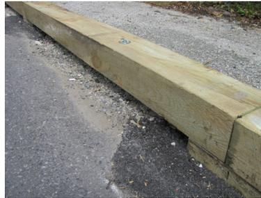
Photo 35. Close-up of timber curb raised to allow for drainage.
