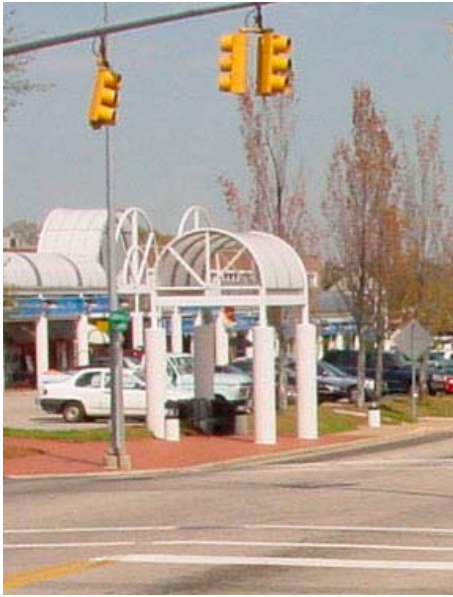
Existing Bus Stop
