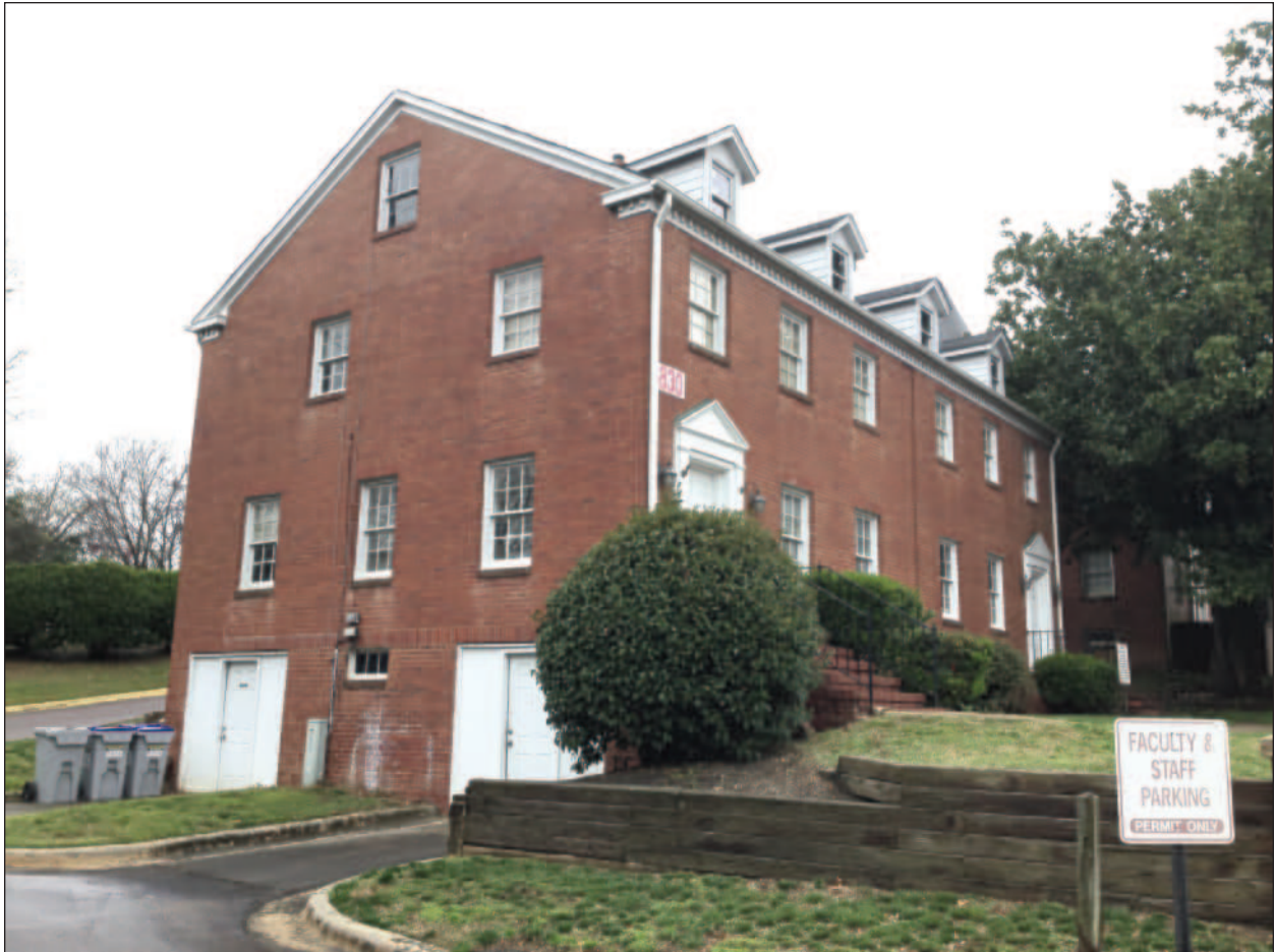
Figure 4.6. Colonial Revival Style Duplex, 830 South Wilmington Street, Facing Northwest
