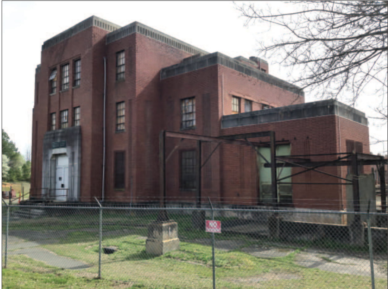
Figure 4.12. Raleigh Water Works and E.B. Bain Water Treatment Plant (WA4179), Facing Southeast
