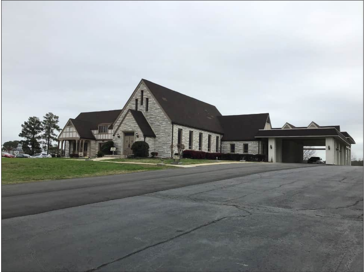
Figure 5.2. Gray Funeral Home, Facing Northeast
