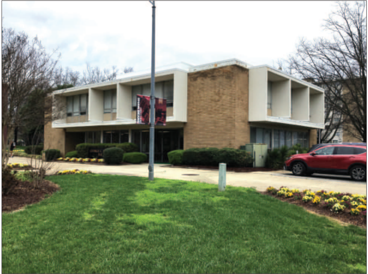
Figure 4.8. Administration Building (WA8073), Facing Northeast
