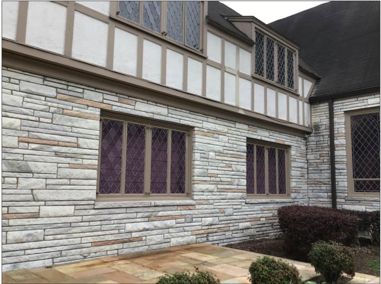
Figure 5.5. Gray Funeral Home, Detail of Windows, Facing Southeast
