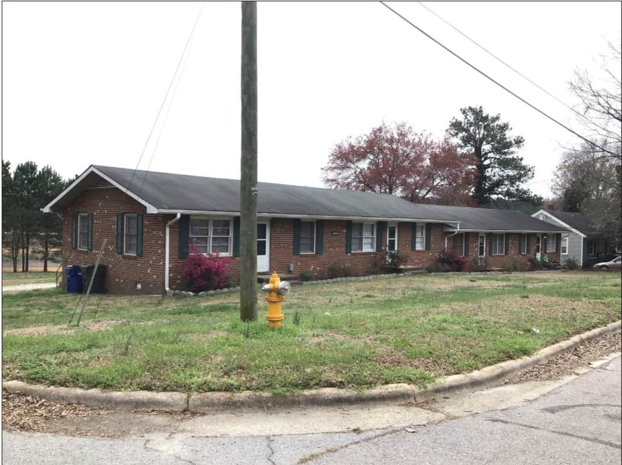
Figure 5.22. Hertford Village, Multi-Family Residence, 2601 Newbold Street
