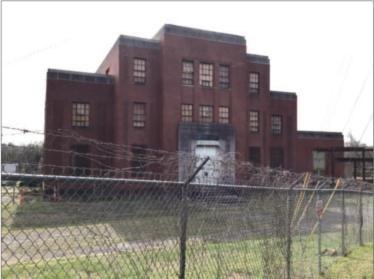
Figure 4.11. Raleigh Water Works and E.B. Bain Water Treatment Plant (WA4179), Facing Southwest
