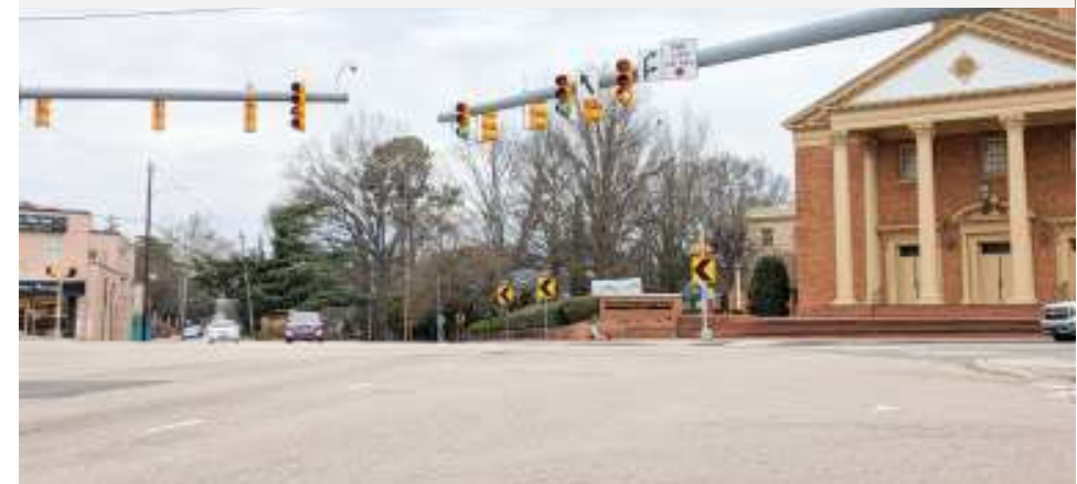
Five Points Intersection Signal Upgrades
