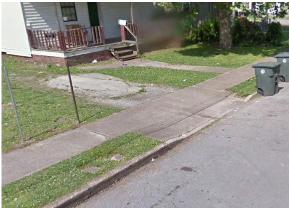
Sidewalk built through a driveway
