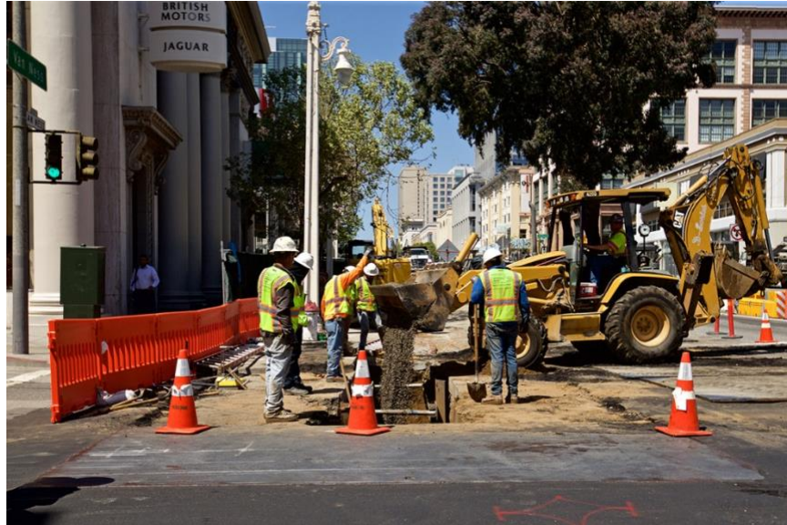
Figure 5.8 BRT Station Construction 20
