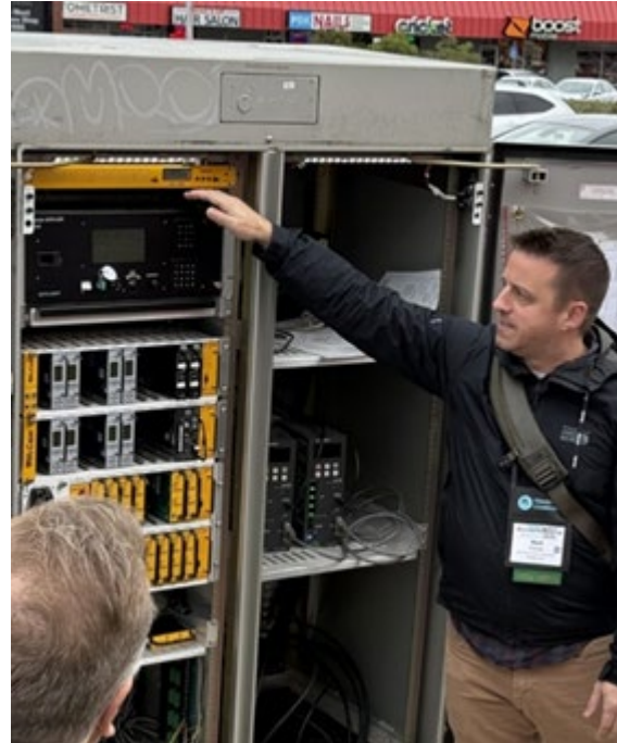
Figure 7 Mark Haines of Portland Bureau of Transportation Explains Traffic Signal Priority for FX2 Bus (image by Patrick McDonough)
