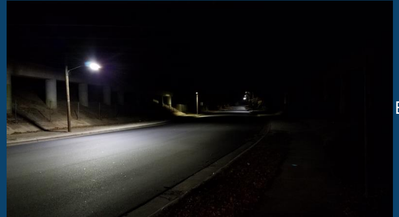
Underpass Lighting: State Street at I-40
